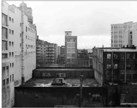
Regal Place Hotel (1909) 144-46 West Hastings Street; Gardiner & Mercer, architects, C-print,2000-2003.
