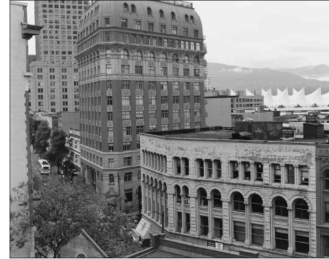
Dominion Building (1908-10) 207 West Hastings Street; J.S. Heyler & Son, architects; and Flack Block (1899) 163 West Hastings Street; William Blackmore, architect, C-print, 2000-2003.
